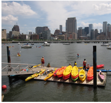
A gangway to a floating dock provides boat access throughout the tidal cycle. Minimizing the number of spud piles fosters free water flow and minimizes sedimentation.
